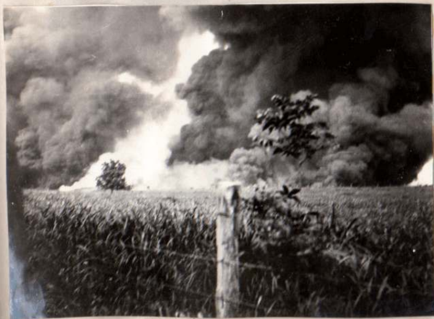
Magnolia tanks afire - Flood
