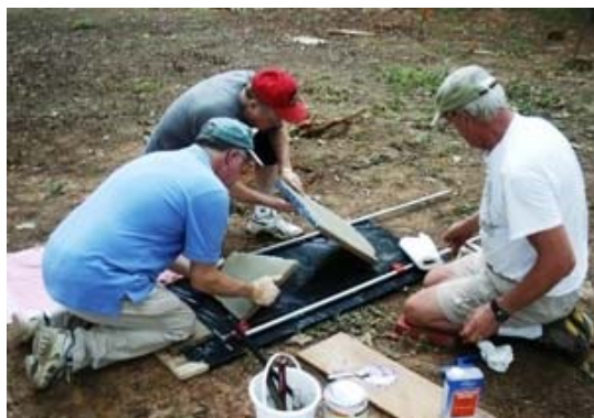
After the broken edges have been cleaned, the pieces are carefully aligned face up on the work surface.
