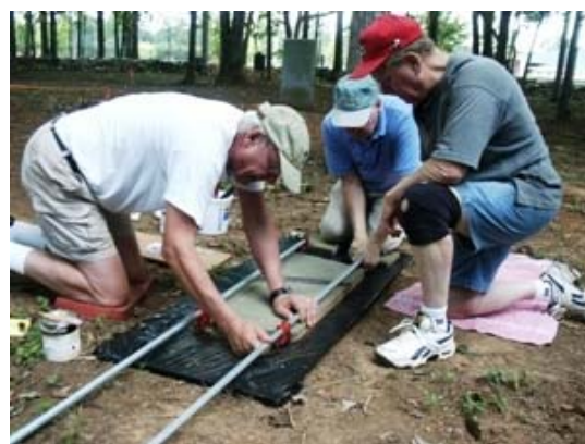
Long pipe clamps are placed on each side of the tombstone and tightened slowly.
