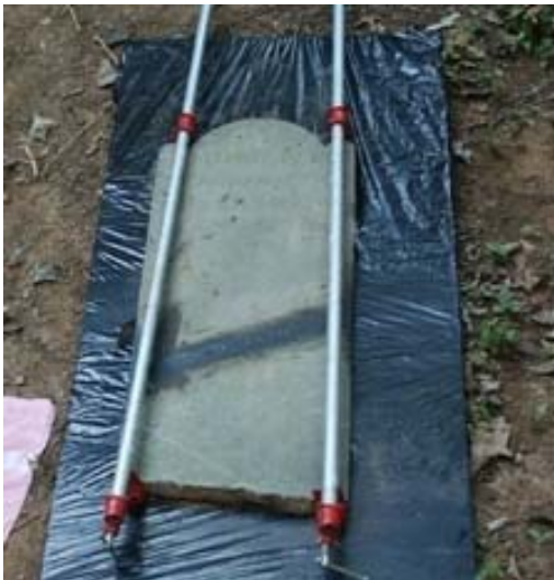
Clamped tightly, the pieces are allowed to dry for several days.
