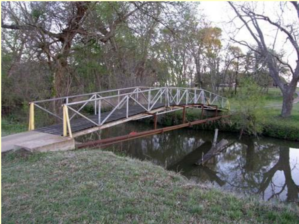
Walk Bridge Photo courtesy Barclay Gibson , March 2008
