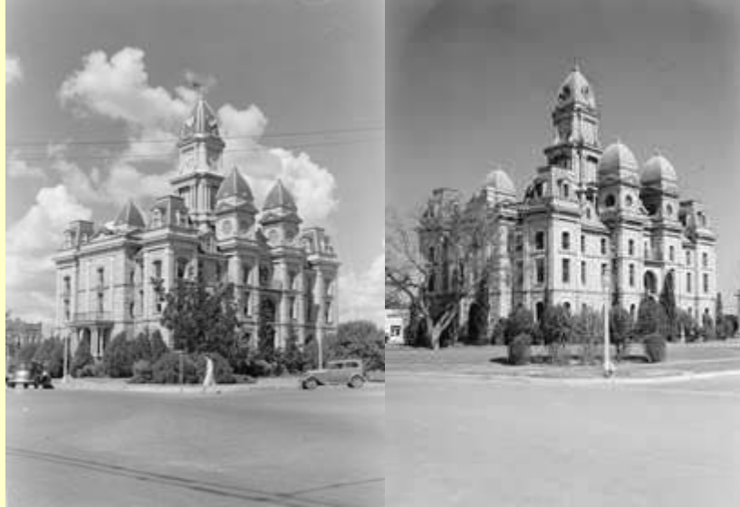
L - Caldwell County Courthouse in Lockhart, Texas R - Goliad County Courthouse in Goliad, Texas 1939 photos courtesy TXDOT
