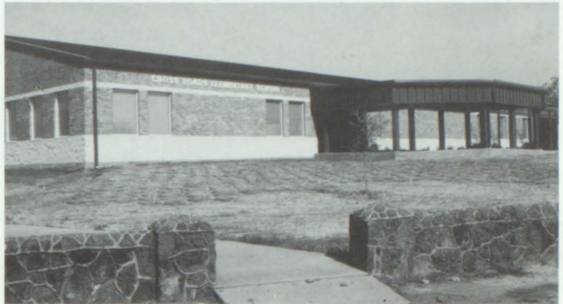
Keeping stone wall in tact provides link with past.
