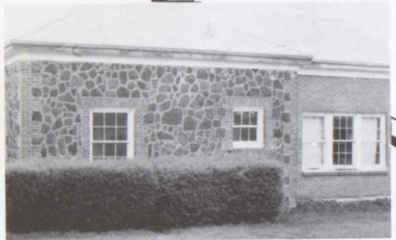
Solid as a rock Brick and stone combine to give the original Homemaking building its earthy appearance.
