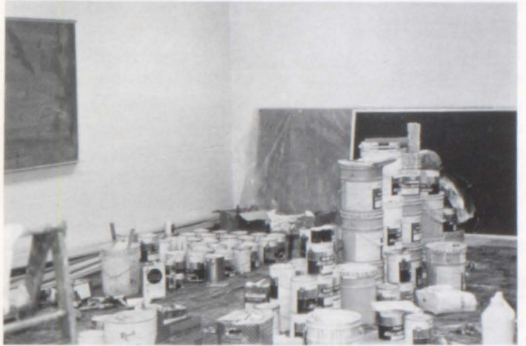
Taking stock Mrs. McKinney's room serves as a paint storehouse shortly before completion.
