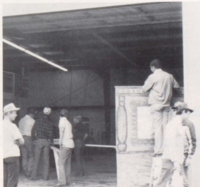
Work at Ag Barn
